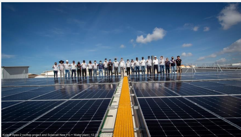
Kidgall Apex-2 rooftop project and Solarcell New PG + Water plant | 12.07.2023
