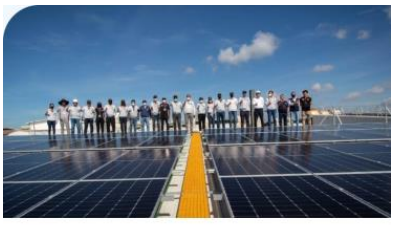
2023.07.14 Apex GREEN Project Part of phase 1 of the Apex Solar Project has been completed ahead of schedul...
