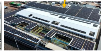
New Water Plant and FG
