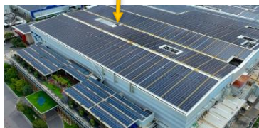
Head Office and Rooftop
