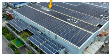
Head Office and Rooftop
