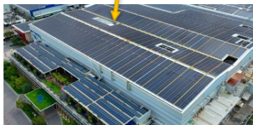
Head Office and Rooftop
