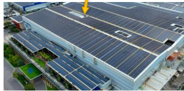
Head Office and Rooftop
