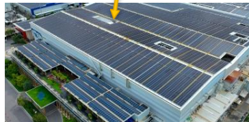
Head Office and Rooftop
